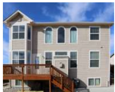
Wood Deck. Full Unfinished Basement Has Garden Level Windows.
