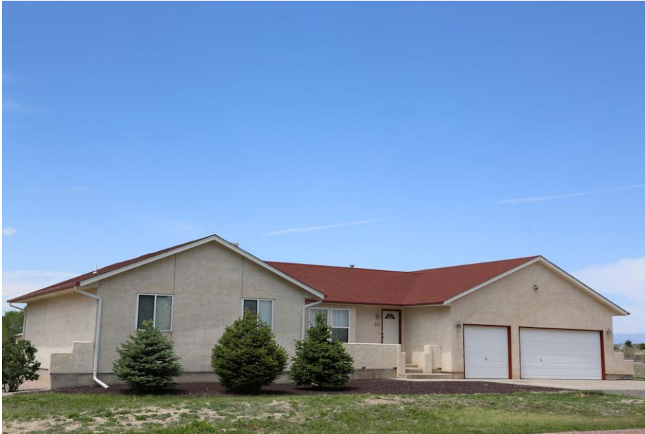
3-Car Attached Insulated Garage. New Roof. New Downspouts.
