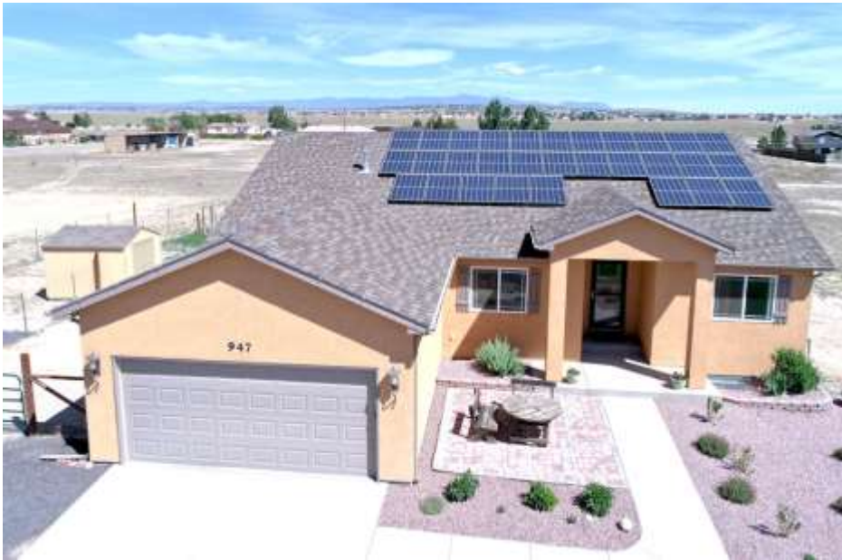
2-Car Attached Garage. View of Pikes Peak. Solar Generation System Is Owned—Not Leased.
